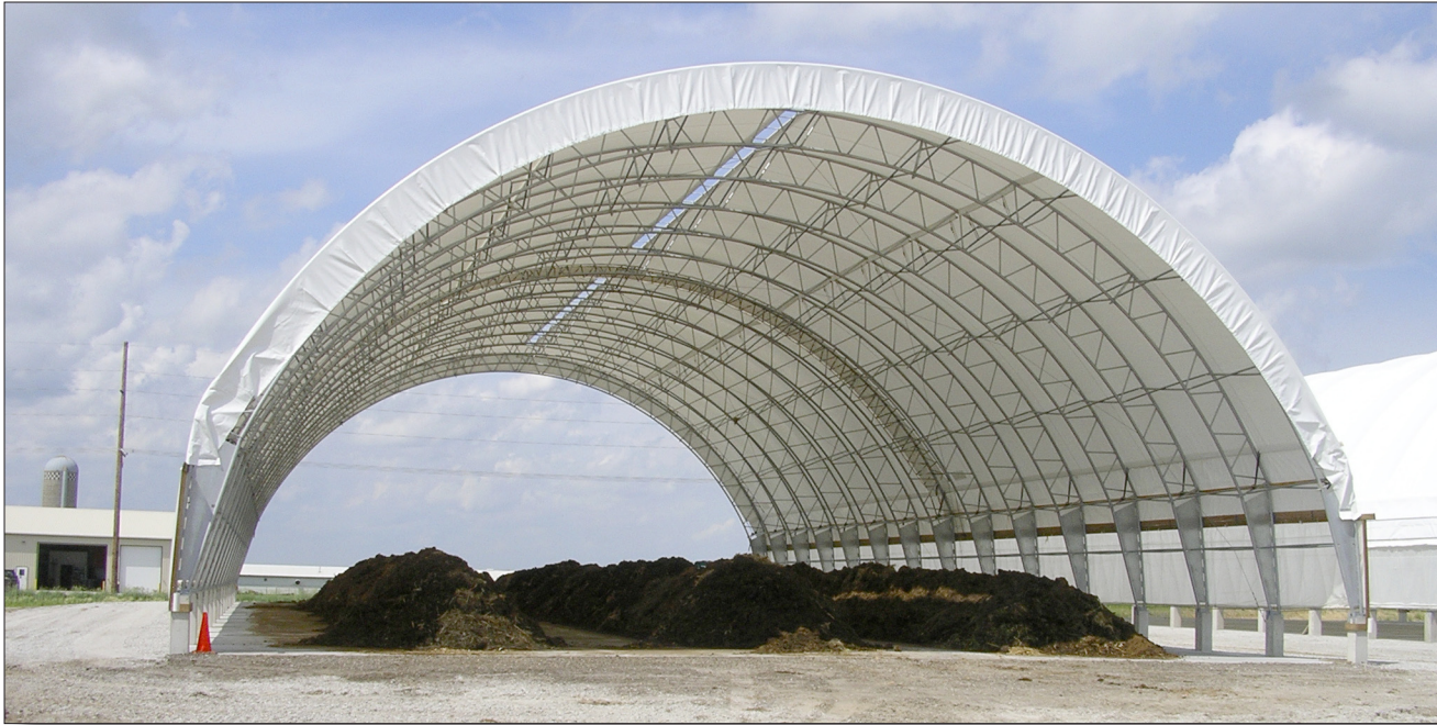
Composting operations occur in large hoop barns to reduce the risk of runoff and leaching.
